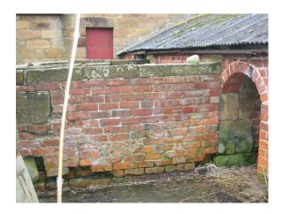
**The Piggeries** These consist of three pigsties each with an enclosed exercise area surrounded by a six foot wall. The walls are pierced with slots for pouring in the swill. The structure shows signs of much rebuilding of brick on stone, the shape however has remained unchanged since it was first depicted in 1856. They show signs of having not been used for a number of years.
