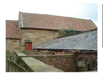
The west barn seen from over the piggeries. Externally both barns fit with mid C18 style but have no precise dating features. The roof trusses which are later with hanging king posts, could be anywhere between 1780 and 1900. Walls are one block thick and buttressed internally. The earliest known single block wall in the area is dated 1740.
