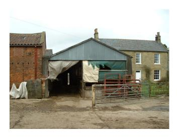
The present end view of south side of the foldyard. Originally described as a line of loose boxes in 1910. It retained its long narrow rectangular shape and was a separate entity until the 1970's, when it was roofed over to cover the space between it and the foldyard. Fabric etc indicate an early 18C date.
