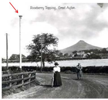
Harry Taylor's scheme called for ventilation stacks at the extreme ends of each leg of the system. The stack on the Guisborough Road can be seen in an old postcard.
