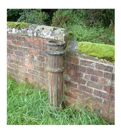
The ventilation stack at the bottom of Station Road has been cut off.
