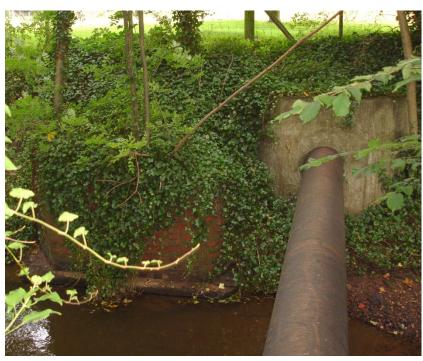
The current crossing of the River Leven is a 1903 replacement for the original pipe, which was swept away in floods. The brick abutment for the original pipe can be seen on the left. Considering the small diameter of the pipe, it is not surprising that the drainage system cannot cope in periods of heavy rainfall.
