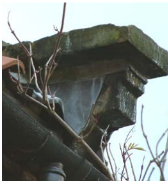
Stone copings at the south gable terminate in decorative, moulded kneelers
