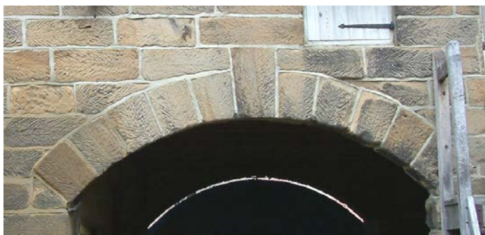
Voussoirs and a keystone, with herringbone tooling evident on the stonework supporting a late 18 th century date.
