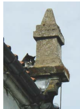
Stone copings at the south gable terminate in decorative, moulded kneelers
