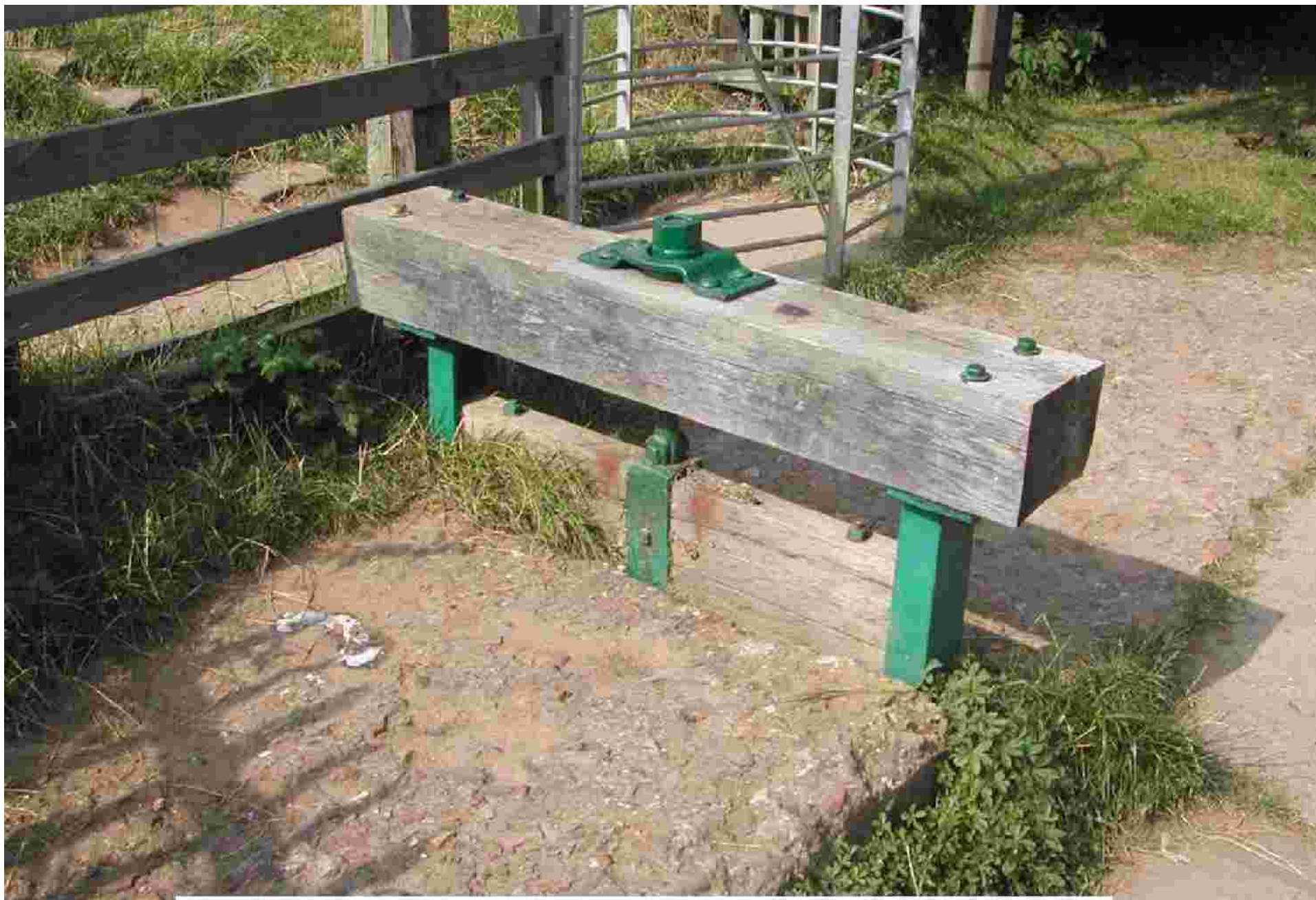
The SLUICE GATE in Waterfall Park– by which water was allowed to flow from above the dam into the mill Race.
