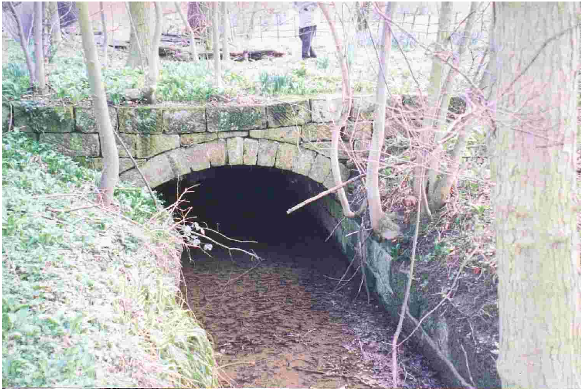
EXIT FROM TAIL RACE CULVERT
