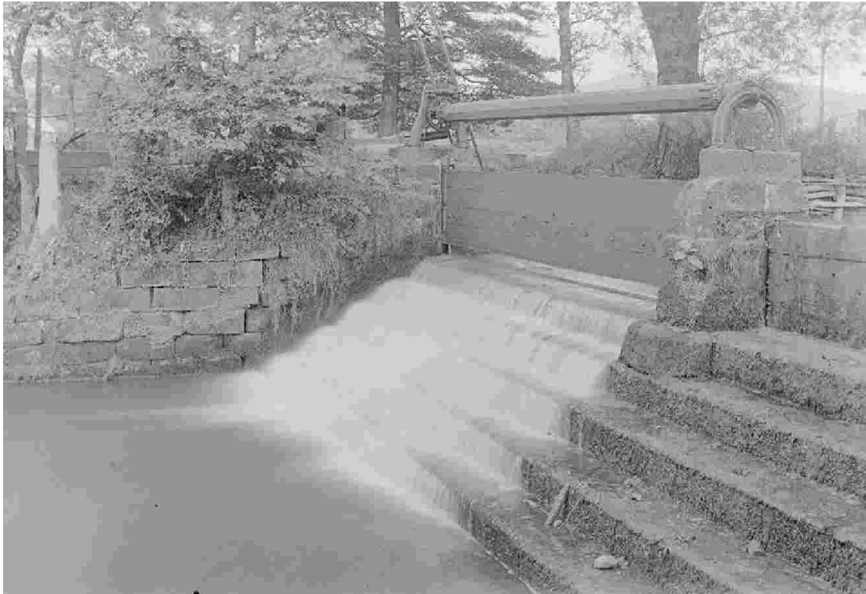
MILL DAM 1936 – The boards (which could be lowered into position) would raise the water level sufficiently to fill the reservoir and also provide adequate head for the working of the mill. The Race was just the other side of the far parapet.
