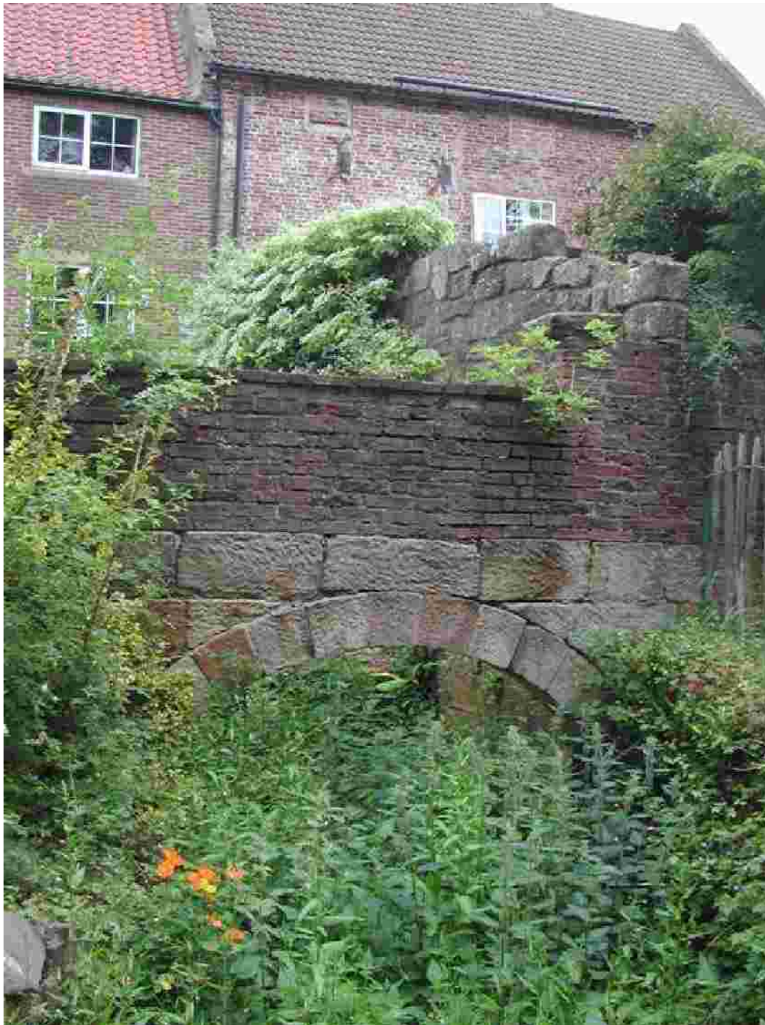
BACK OF GRANGE MILL – THIS ARCH WAS WHERE THE 'TAIL RACE' EMERGED FROM UNDER THE LARGE REAR EXTENSION WHICH WAS IN USE WHEN IT WAS AN OIL MILL
