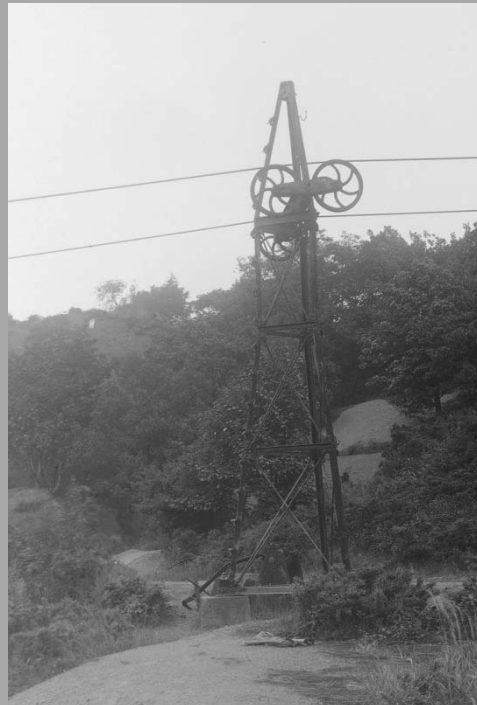
One of the supports for the aerial ropeway from the Ayton Banks Ironstone Mine , through Cliff Rigg Woods to the main line sidings
